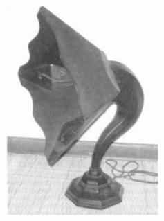
Master horn speaker, that fit over a nub on the neck. There actually are two sets of slots in the flange so you could either orient the bell so it is flat on the top, or tilt it with a pointed end on top.
