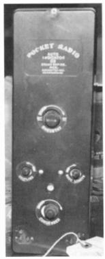
The Pocket Radio, manufactured by the Auto Indicator Co., measures 4" x 12" x 2" deep. The four controls are labeled "Rheostat," "Coupling," "Wavelength," and "Condenser." In good condition, except for a chip in the case, it sold for \$225.
