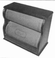
DICTOGRAND ROLL SPEAKER – This unusual paper cone speaker was manufactured by Dictograph Products Corp., 220 West 42nd St., New York City. It measures 13½" x 6¾" x 11¼". The Dictogrand reproducer is connected at the center fold of the two paper rolls and has an adjustment screw out the back. The rather thick, parchment-type paper has a gray-brown, mottled finish, and the lettering and edges are embossed. The unit sold for \$16.50 in 1925. (Wally Worth – Wollaston, MA)
