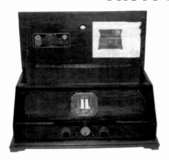
RCA RADIOLA MODEL 25 – This 6-tube receiver is battery-powered and operates with five Type UX-199 tubes and one Type UX-120 output tube. Manufactured by Radio Corporation of America in 1925, it sold, with tubes, for \$165. The company produced over 94,000 units of this receiver. (Clark Trissell – Lincoln, NE)
