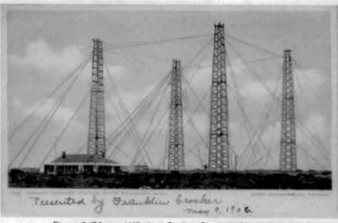
Figure 6. "Marconi Wireless Station, South Wellfleet, Mass." (1906) The tower quy wires are clearly visible in this card.
