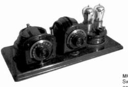
ATWATER KENT TYPE 3925 – This 1925 bread-board receiver is sometimes called the Model 1, for it was the first of this type of Atwater Kent board receivers. On the left is a coupled circuit tuner; in the middle, (installed only by the local dealer), is a variometer to make it regenerative; at right is a 2-tube TA unit, all mounted on a mahogany board. This set sold for \$32, without the variometer, and \$42 complete, without tubes. (Dave Crocker – Mashpee, MA)
