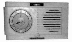
GE MODEL 501 – This ivory plastic clock radio was manufactured in 1950 by General Electric. It tunes AM only and uses three miniature and two octal tubes as follows: (1) 50C5, (1) 35W4, (1) 12BA6, (1) 12SQ7, and (1) 12SA7. (Loren P Ashworth – New Paris, OH)
