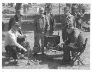
Tom Horsfall's SCR-284 field set, powered by a hand-cranked generator, is in full operation.
