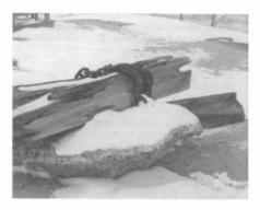
One of two remaining 10-foot sections of wooden tower beams, bolted and chained to concrete footings.
