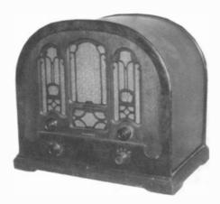
ATWATER KENT MODEL 708 – This 8-tube cathedral was manufactured in 1933 by the Atwater Kent Manufacturing Co. of Philadelphia, Pennsylvania. It measures 12½ high and 16" wide. The dial appears behind a small window opening at the right. (Wally Worth – Wollaston, MA)
