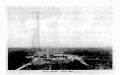
"Radio Station, Rocky Point, L.I." This is RCA's "Radio Central" which went on the air on November 5, 1921, as the Riverhead Facility. The antenna towers were 412 feet high with 150 feet cross arms. The last tower was demolished on December 13, 1977.
