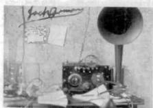
Figure 2. The receiving setup is similar to that shown in Figure 1, except that the left-hand tuning dial of the receiver has been changed from a vemier type to a direct-drive dlal. This photograph is also dated "1929.
