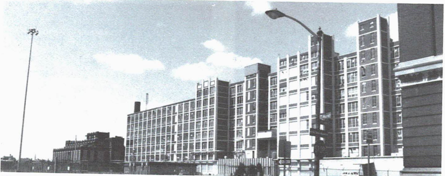
Figure 5. This photo ran in our November 1994 A.R.C. with the caption: "These other 'old' GE/RCA/VTMC buildings in Camden are likely targets for demolition..." As reported in the Rouse article, two of them bit the dust in 1997. Three others were imploded in 1995. (Photo courtesy of Chris Russo.)
