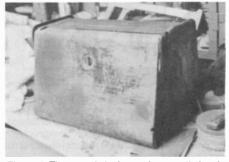
Figure 4. The use of glazing and spot putty levels the surface after the old covering is removed.
