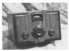
Figure 2. Front view of the Magnavox Eton Model T, ca. 1927, made to slide into a cabinet, which is missing.
