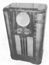
NORTHERN ELECTRIC MODEL 1121A – This 11-tube Canadian radio tunes the BC band, the police band, and 3 SW bands. It features bandspread tuning on the SW bands and AFC on the BC band. A "fidelity control switch" controls the selectivity of the two IF stages. (Marcel La Bossiere – Marmora, Ontario, Canada)
