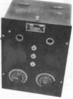
CLARIPHONE MODEL UN-KNOWN - These detector (left) and amplifier (right) units were made by Campbell Electric Co. in Lynn, Mass., probably in 1922. According to the Lynn Historical Society, Campbell made electric and magnetic apparatus. Campbell's radios appear to be very rare. Any others? (Merrill Bancroft - Townsend, MA)
