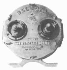
**BELL GAP** – Manufactured by the Electric Machine Co. of Indianapolis, Indiana, this rotary spark gap, ca. 1920, has an aluminum housing. (Larry Chestnut – Ellington, CT)
