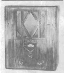
FADA MODEL 73 – This 1933 Fada tombstone features a 7-tube broadcast band chassis with phono input. The cabinet is basically a plain rectangular wooden box. However, by adding Art Deco stair-stepped routing, toning lacquer and book-matched veneer, this radio takes on a more expensive appearance. (Robert Bailey – Jacksonville, FL)
