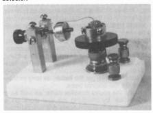
Figure 5. The Duck Type G crystal detector.
