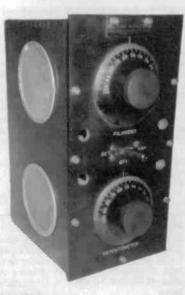
SPARTON MODEL 610 – A TRF design of simple yet sturdy construction, this set has 5 stages of RF amplification giving good performance on weak signals. Three separate chassis house the tuning condenser, RF stages and power amplifier. (Greg Jones – Westerly, RI)
