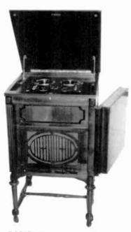
RCA RADIOLA AR-813 – This 6-tube catacomb superheterodyne radio, circa 1924, has the same circuit as the Super VIII (AR-810) and the portable AR-812. The radio is factory installed in a nice cabinet with a built-in horn, a loop antenna in the front door, room for batteries inside the cabinet, and tube access through a removable panel above the horn opening grille. (Joe Urbanovitch – Sylmar, CA)
