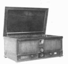
**STROMBERG-CARLSON 635A** - This 7tube electric set has excellent shielding. It receives twenty stations utilizing its Model 11 wall speaker. The set has had no repairs; all parts are original from 1928. (Walter Worth -Wollaston, MA)
