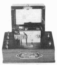
BROWN MICROPHONE AMPLIFIER - This is a one-stage microphone amplifier made by S. G. Brown Ltd. in 1923. It was designed so that several pairs of headphones could be used from a single crystal set. (Erwin Macho -Vienna, Austria)
