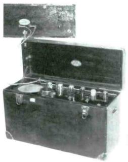
GLED PORTABLE - Six Type 199 tubes were used in this 1925 receiver by Gled Radio Co. of Philadelphia. The insert containing the loop is stored in the lid and is supported by brass rods in the open cover. It has a built-in speaker and room for batteries with an access door in the rear. (Walter Worth - Wollaston, MA)
