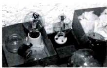
The 1908 DeForest spherical audion. Despite the open filament and broken grid and plate leads, it brought a price of \$185. It is surrounded by an assortment of old light bulbs and sockets.
