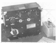
3-tube aircraft radio receiver, Model SCR-59, 1917-18, non-regenerative detector and two-stages of audio amplification. (George Potter)
