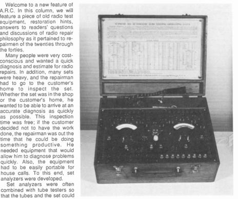
provision for external prods so that the analyzer could also be used as a multimeter for more measurements of voltage, current, resistance, and continuity. The analyzer, combined with a tube tester, allowed the repairman to find almost any problem, often without having to remove the chassis from the set. This made the job of the serviceman much quicker and easier.
