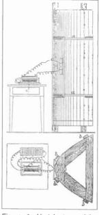
diameter; the Figure 1. Hertz's transmitting other end was apparatus and parabolic mirror.
