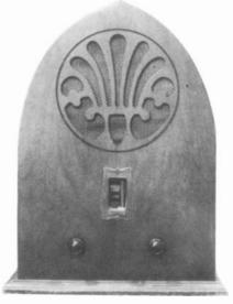
SIMPLEX MODEL H - Manufactured by the Simplex Radio Co. of Sandusky, Ohio. Introduced in 1930, it was Simplex's first mantel radio. Selling for \$69.50, it was also available in a striking ebony and silver modernistic cabinet. Simplex radios were sold under many brand names. (Frank Heathcote, Logansport, IN)
