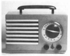
seven-tube AC-DC. the Aristocrat. Its tuning range is 540-1630 kc. (standard American broadcast and police). Some of the early Emerson midget sets had wooden cabinets; others were made of paper-covered cardboard which looked like leather in grain and texture. These receivers have a built-in loop antenna and work best with the rear of the set pointed in the general direction of the transmitting station.
