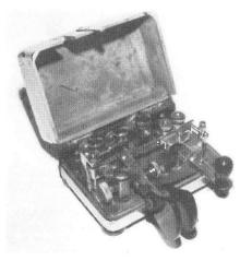
THE ULTIMATE - This "flip top" bug was made for the traveling telegrapher who would take it with him to sporting events, etc. and drop it in his pocket when finished. Patented in 1925, this model was made of cast bronze. Some of the later models were made of the "infamous" pot metal and didn't survive. A real "gem", I paid \$3 for it about 20 years ago.
