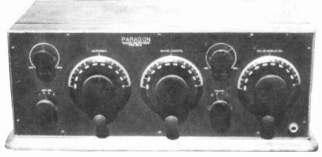
PARAGON - Model RB-2, a 3-tube regenerative receiver introduced in 1924 by Adams-Morgan Co. An unique feature of most RB-2's was the ability to switch tube filament voltage via plug jumpers behind each tube. This jumper allowed a person to use various tubes. (Craig Huseboe - Marshalltown, IA)
