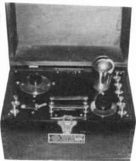
SPLENDID DELUXE - One tube radio receiver, it uses a 201A tube. Type "B" is in a box type cabinet 10" wide, 8" high, and 7" deep. Manufactured by W.F. Mains Radiophone Co. of Cedar Rapids, Iowa, and Chicago, Ilinois. (David McKenzie - Eustis, FL)
