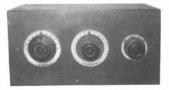
CUTTING & WASHINGTON - Type 15, this receiver uses one 99 type tube. Room inside the cabinet for the 22.5 volt "B" battery. (R.A. Hostler - Findlay, OH)
