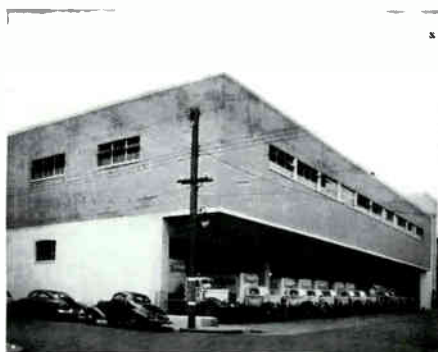
Cantilever loading platform building Orange, N. J. Brewery.
