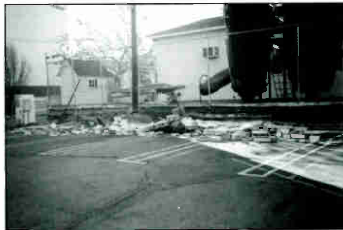
The remains of a retaining wall that surrounded a Sherman Oaks pre-school.
