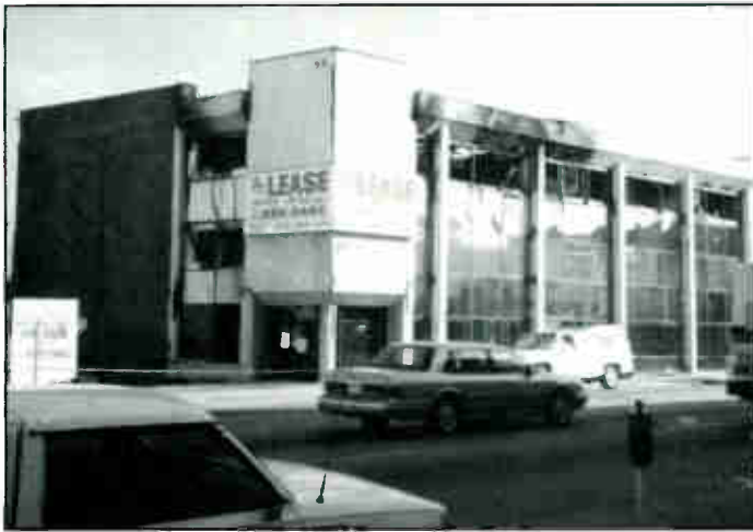
Ventura Blvd. looked something like Beirut after the 6.6 quake rumbled through.
