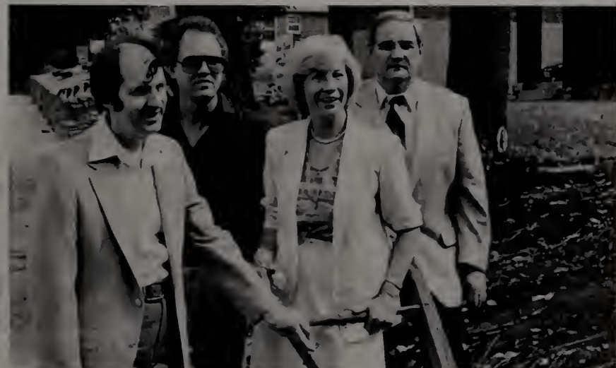
BREAKING NEW GROUND — Jack McFadden broke ground recently for his companies, McFadden & Assoc., Inc. and McFadden Artist Corp., new office building which will be located at 818 18th Ave., South. Pictured (l-r) are: Billy Deaton, local talent director; Jackson Brumley, Frizzell & West's manager; Jo Walker-Meador, director of the CMA and McFadden.
