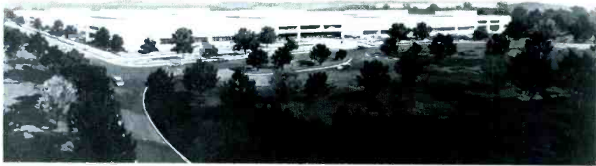
FUTURE HOME — Sega Enterprises, Inc. plans a major expansion of manufacturing facilities of its Gremlin Industries division that produces computer video games. Sega has signed a lease agreement to occupy this 123,200-square-foot building in the Rancho Bernardo Technology Park in north San Diego, which will employ approximately 500 people. Occupancy is scheduled for mid-September of this year.
