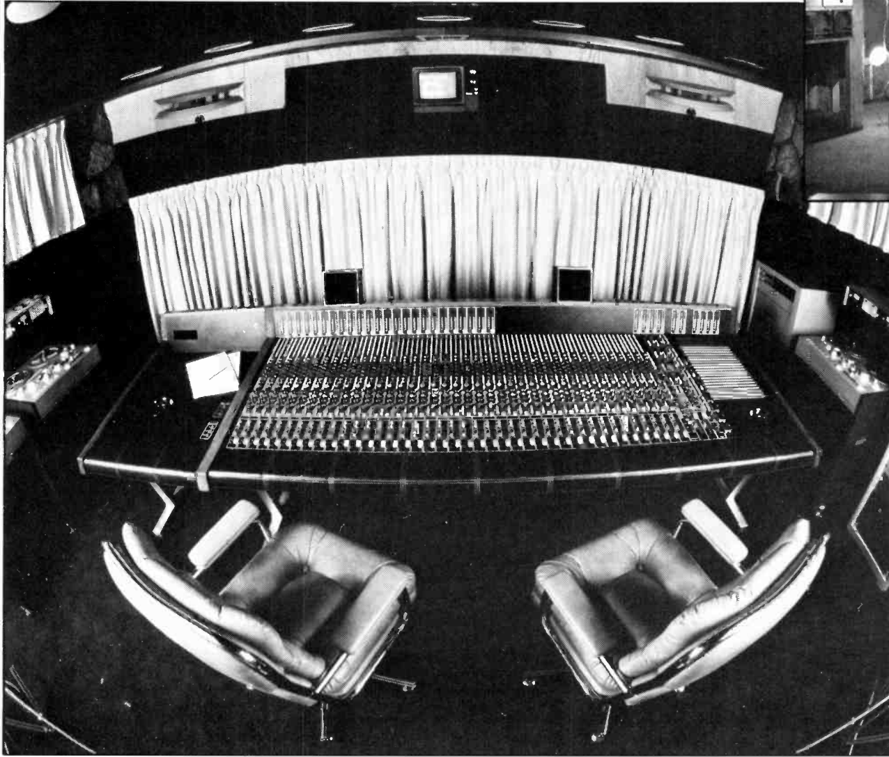
Sounds Interchange in Toronto: The solution was to sink the studio five or six feet below the old floor level, so the new control room could overlook it and maximize space. Says manager McCluskey, "With the new rooms, bands can finish the mix a lot faster. We can move people through the studio faster, too, by shifting them into the new small studio for finishing up."
