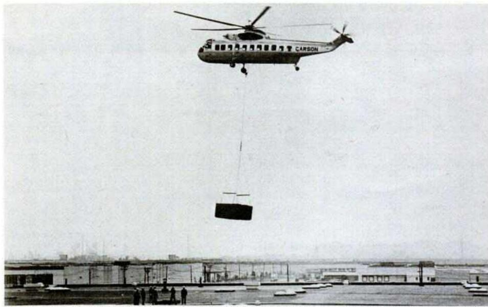
AUDIO AIRLIFT—Construction engineers use a helicopter to position a giant air-conditioning unit in the middle of 12acre roof of new Panasonic distribution center in the Hackensack, N.J. meadowlands. The \$50 million complex is reported on schedule and Panasonic plans to move its warehouses and sales staff to new location by Sept. 1. Administrative staff will shift from New York's Pan Am building by next January.
