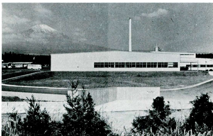
NEW TMI PLANT AT GOTEMBA
