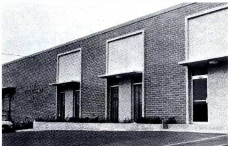
IMMENSE SIZE of the new H. B. Hutchinson Jr. bulk vending distributing complex is illustrated in this photo of the 31,000-square-foot facility in Atlanta.
