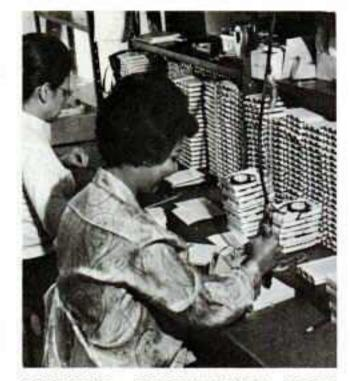
SPLICING CONTINUOUS LOOP tape and sealing the cartridges and cassettes is handled by a separate staff.
