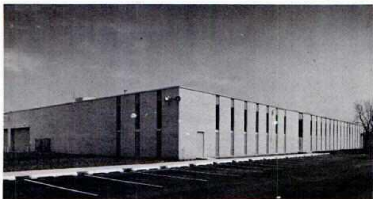
D. GOTTLIEB & CO. has been celebrating its 40th anniversary by moving part of its operation into this new plant at 165 West Lake Street, Northlake, Ill. The firm has occupied three plants in Chicago since Dave Gottlieb founded the firm in 1927.
