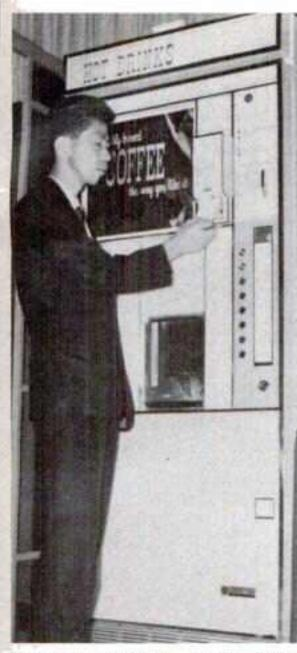
TOSHIO TANAKA, representing Taleisi Electronics Co., the Japanese firm which developed a credit-card-actuated concept for vending machines, inserts card in Rowe coffee machine.
