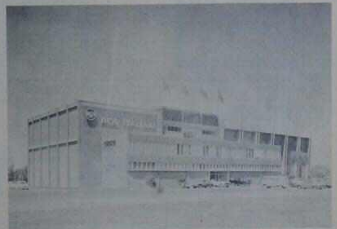
International Facilities. Picture courtesy RCA Italiana.
