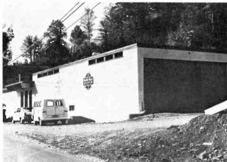
GENERAL VIEW of the newly completed, three-level Black Hills Novelty building shows the ample space the firm now has for its coverage of Western South Dakota.
