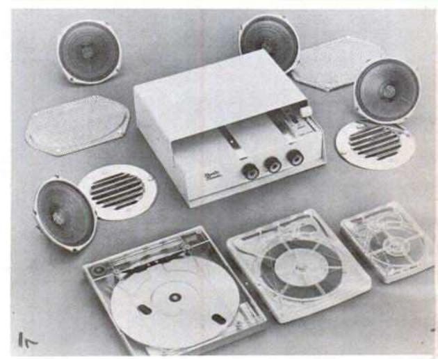
COMPONENTS OF MUNTZ Autostereo car unit, showing tape playback (operates on car battery), two five-inch speakers, with upholstery-matching grille cloth covers for mounting in front, and two five-inch speakers for rear installation. Three different sizes available in perpetual-play cartridge, contains four LP's. Playback lists at \$129.95 plus \$25 for installation and speakers.
