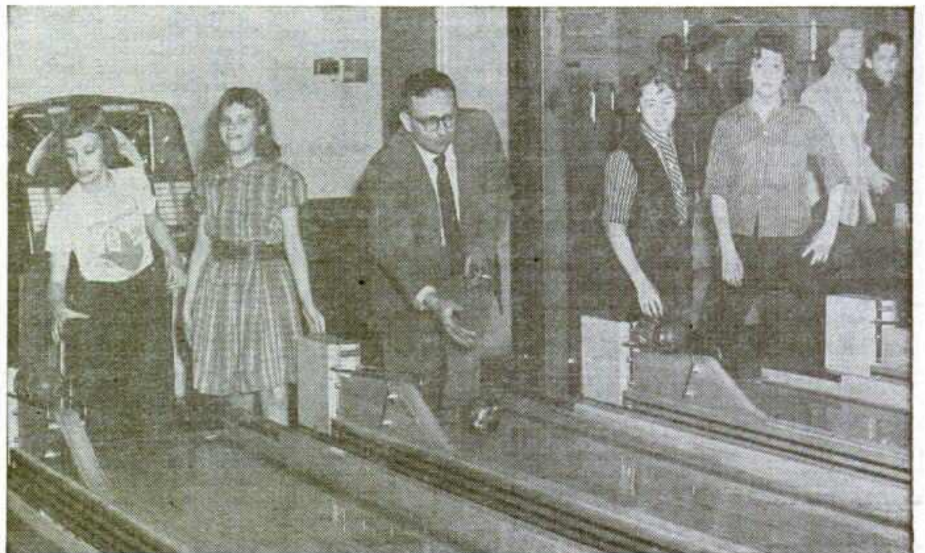
INSIDE VIEW of the Bowl-O-Fun shows William McKenna, the owner (center), giving his young lady customers a demonstration on the alleys. McKenna, a restaurateur, got interested in the bowling set-up as an added attraction to his drive-in set-up.
