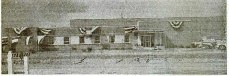
Front and sides of the office section of the combined office-factory are of enameled-face brick. Exterior of remaining portion of the huge structure is of concrete block. The entire 10-acre plant is fenced with a seven-foot-high chain link fence, topped by three strands of barbed wire.
