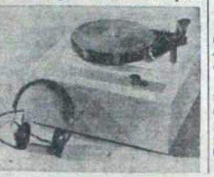
Garrard player with Electro-Voice on Sonotone stereo oartridge and a Clevite "Walco" cartridge. The Clevite "Brush" headphones also serve to cut off any distracting noises in the store situation.
